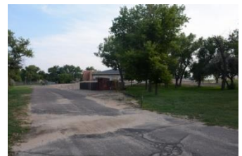
Figure JJ. Lamar Canal, part of Lamar’s storm water collection system (top); east access road drains off to Willow Creek to its east (bottom).
