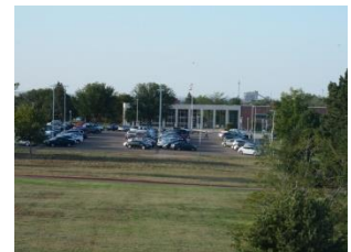
View of the parking facing Bowman Administration Building.
